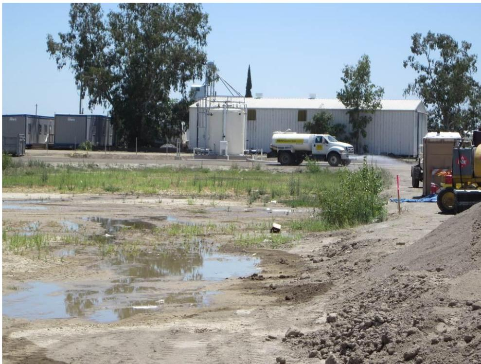
**Photo 3:** On-site dust at the Compressor Station site was being controlled via the use of water trucks.
