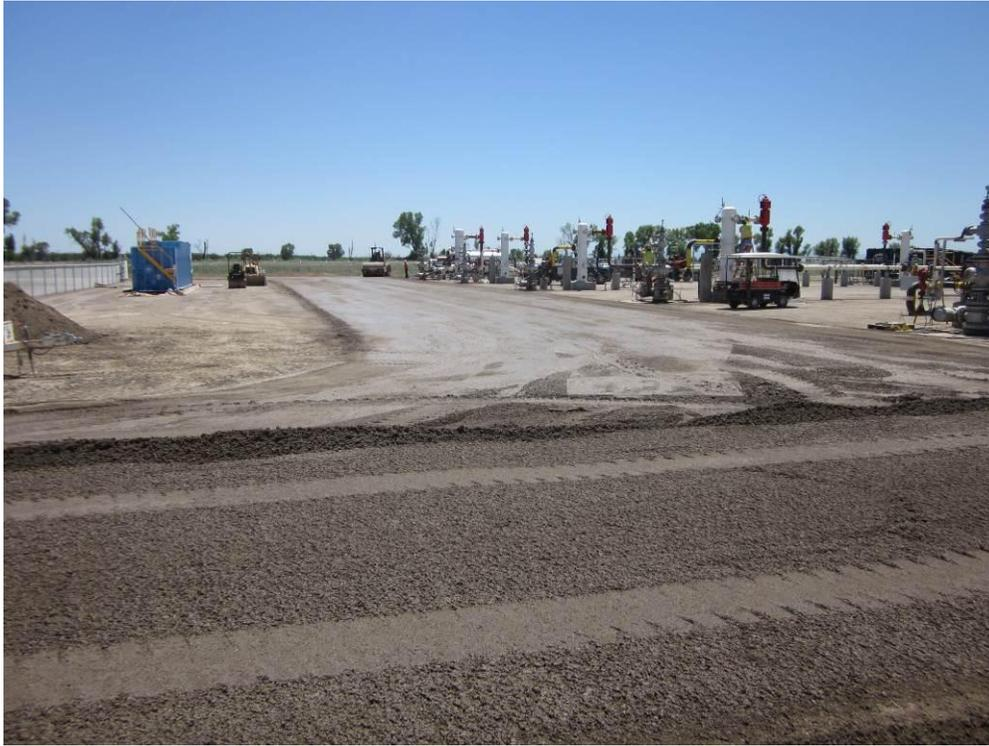
**Photo 1:** The Remote Well Pad site has been graded and installation/rolling of final base material was underway.
